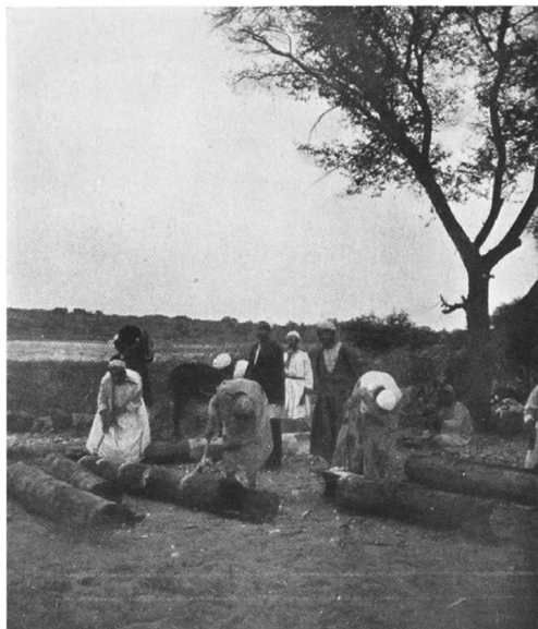
WOODEN PIPES FOR ARTESIAN WELLS, DAKHLA OASIS: SUNT TREE ON RIGHT
