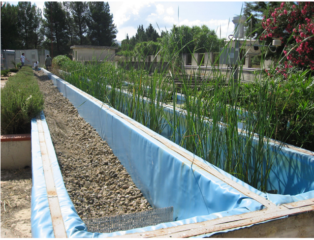
Fig. 2. A view of HSSF pilot system located downhill from the sewage plant in Piana degli albanesi (Sicily, Italy).
