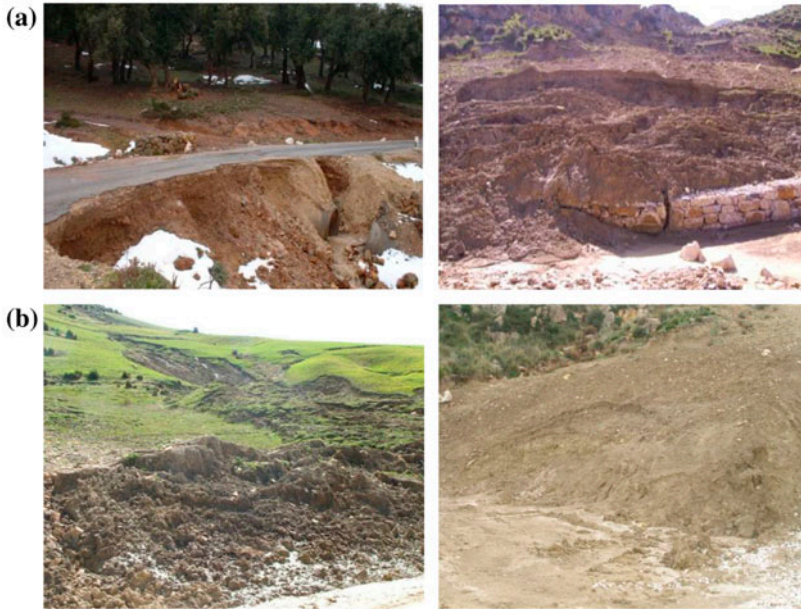
Photo 1. (a) Shallow failures causing damages in the road, (b) Collapse of the clay soil during a period of wetting season [a] (date: 16/03/2006), Local slope failure after the first rainfall episode [b] (date: 20/12/2006).
