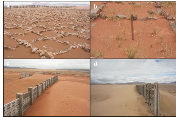
Fig. 11 Photographs of stone checkerboard barriers (SCBs) and sand fences (SFs). a and d in Cuona Lake; b and c in Honglianghe
