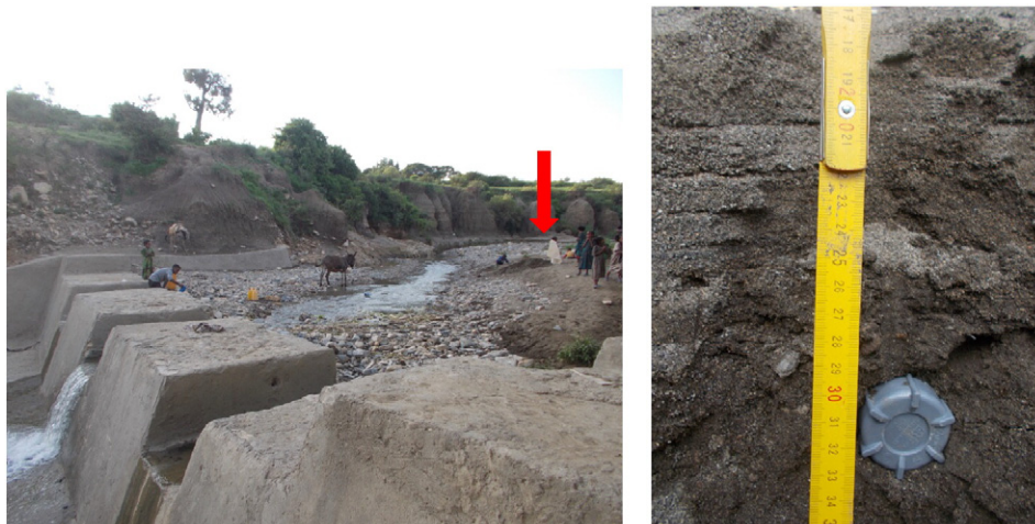
Fig. 3. Sampling site (indicated with red arrow) and sampling of the modern sample (M), just upstream of a newly built check dam in the May Tsimble channel.
