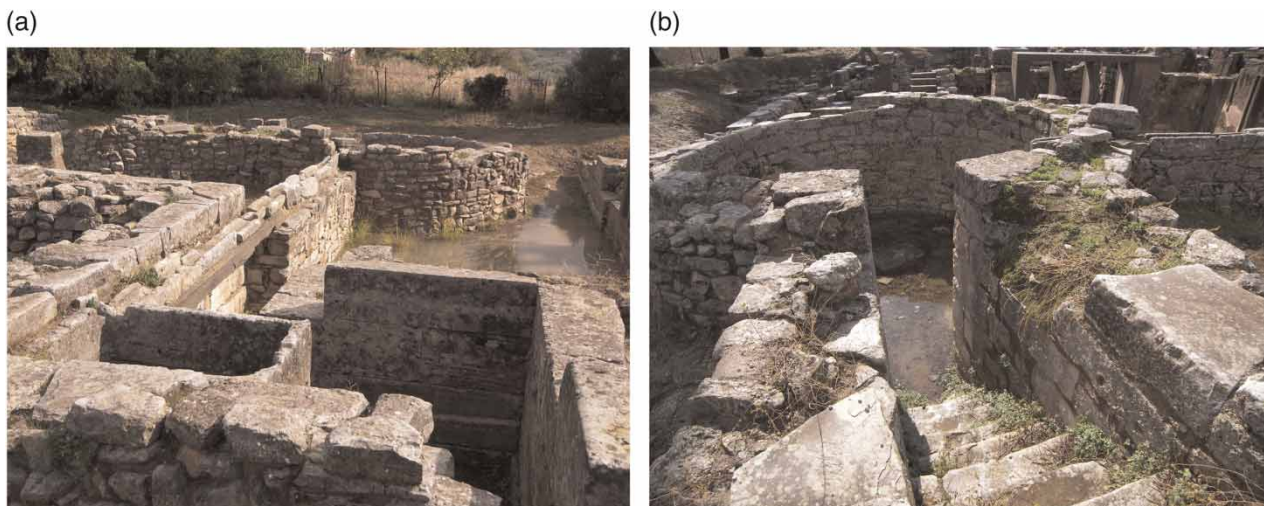
Figure 2 | Cistern in Tylissos, Crete. (a) Sedimentation tank in foreground with stone channel connecting to cistern. (b) Steps leading down to cistern (photo copyright by L.W. Mays).
