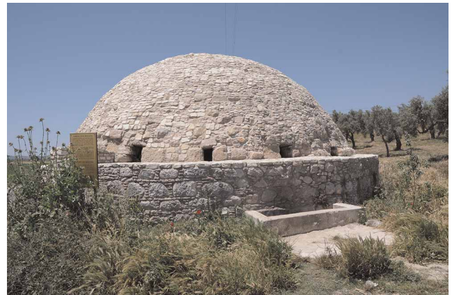
Figure 12 | Ottoman cistern built for military purposes of the Ottoman Army, located near Bodrum, Turkey (photo copyright by L.W. Mays).
