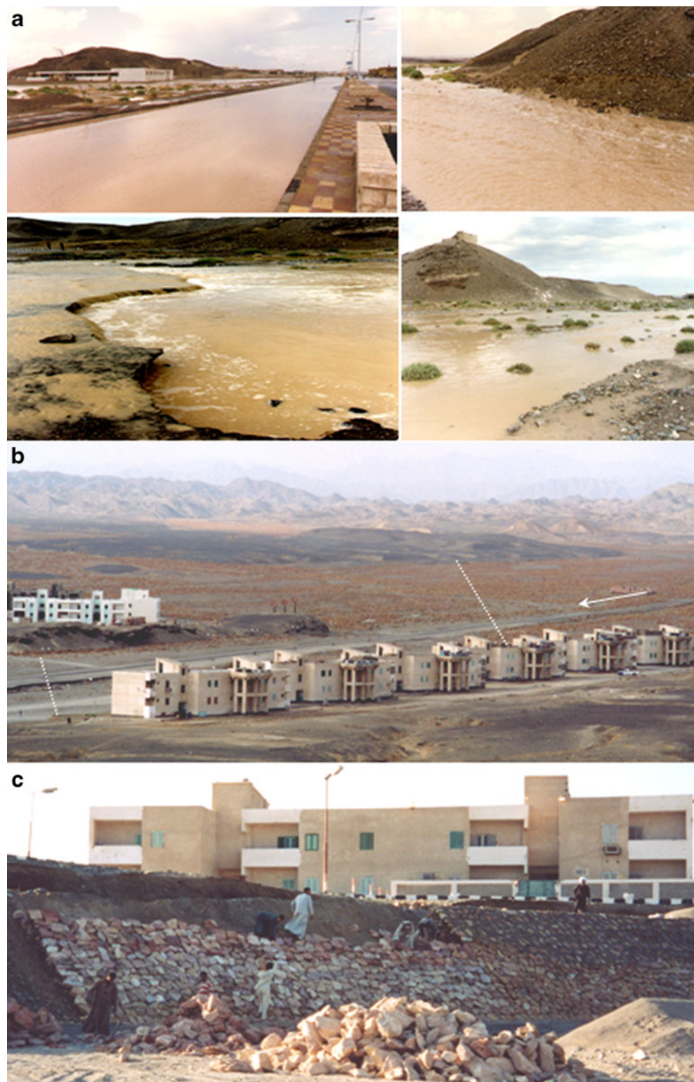
Fig. 3 a Four field photos taken 2 h after a major rainstorm that occurred in 1996. They show a damaged sector of the coastal highway by the flood water ( left, top, and bottom ) and flood water in the downstream area of wadi El-Alam Basin ( right, top, and bottom ). b The narrow channel at the outlet of wadi El-Alam Basin. c Local residents using rocky boulders to strengthen the hillside of the dry river at the downstream area
